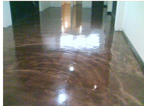
Commercial office floor
