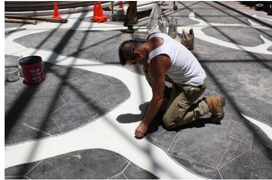
Laying epoxy coating over laser lights in floor motif
