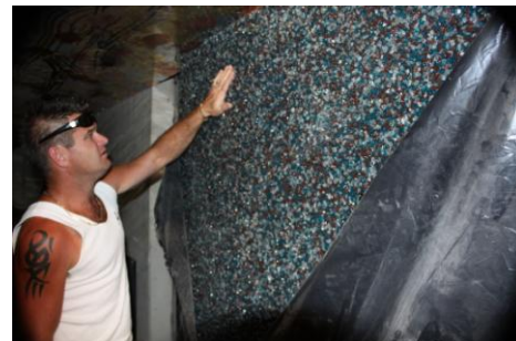
Epoxy and coloured stones in wall feature 'Cloudland', Katarzyna Group
