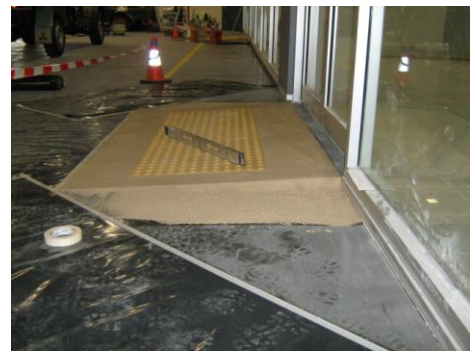
Ramping of step to Office
